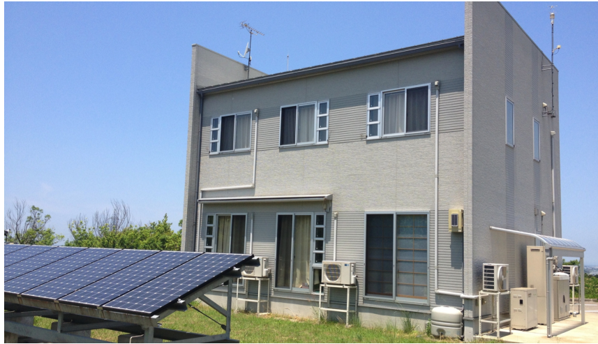
Figure 7.10: A picture of the iHouse, an experimental smart house
