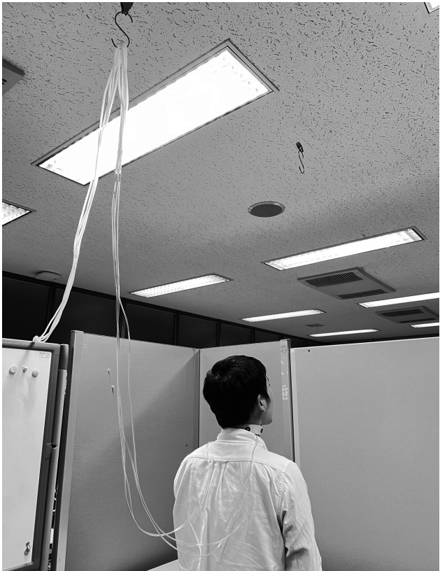
Fig. 5.22 Silicon tubes suspended from the ceiling.
