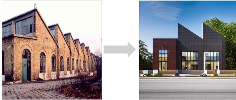
(b) Architectural Renovation
