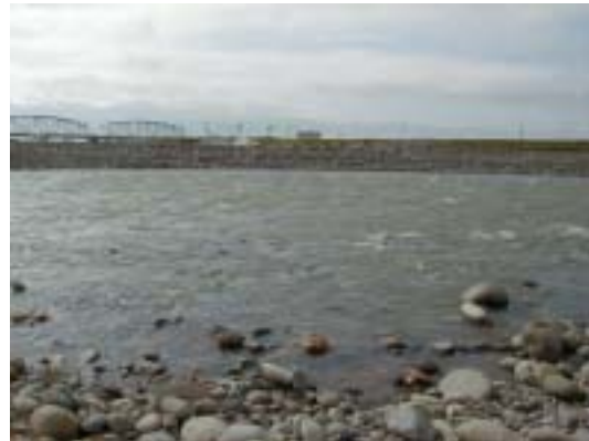
Figure 4.21: Tatsukuchi-bridge on Tedoririver.
